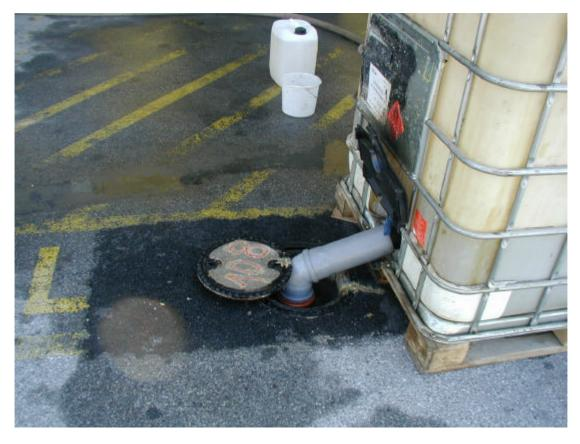
Bioversal 1 % solution is injected into a well:
